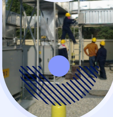
Hvac Duct Installation
